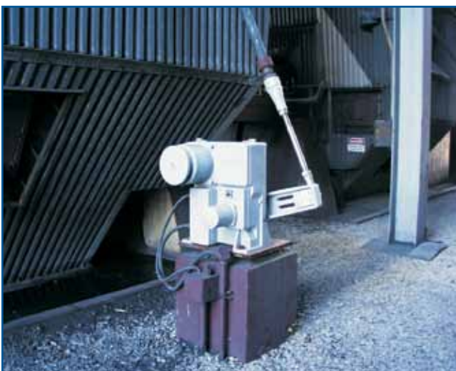
Beck Group 22 drive installed on a damper.
